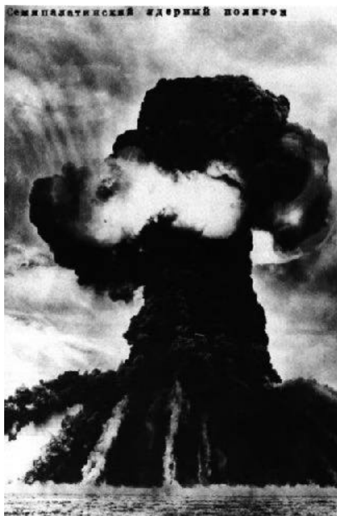
Figure 9. The Soviet nuclear explosion, “Shagan,” of 15 January 1965, designed to create a crater and dam a water reservoir.
